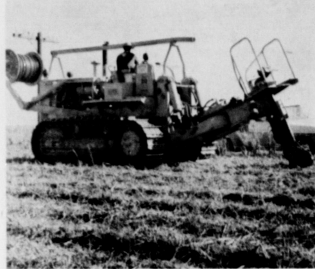
BURYING CABLE FOR GENERAL TELEPHONE ON FM Road 2901. This cable burying equipment slices through the soil, places its cable 36 inches deep, and covers all in one process.
