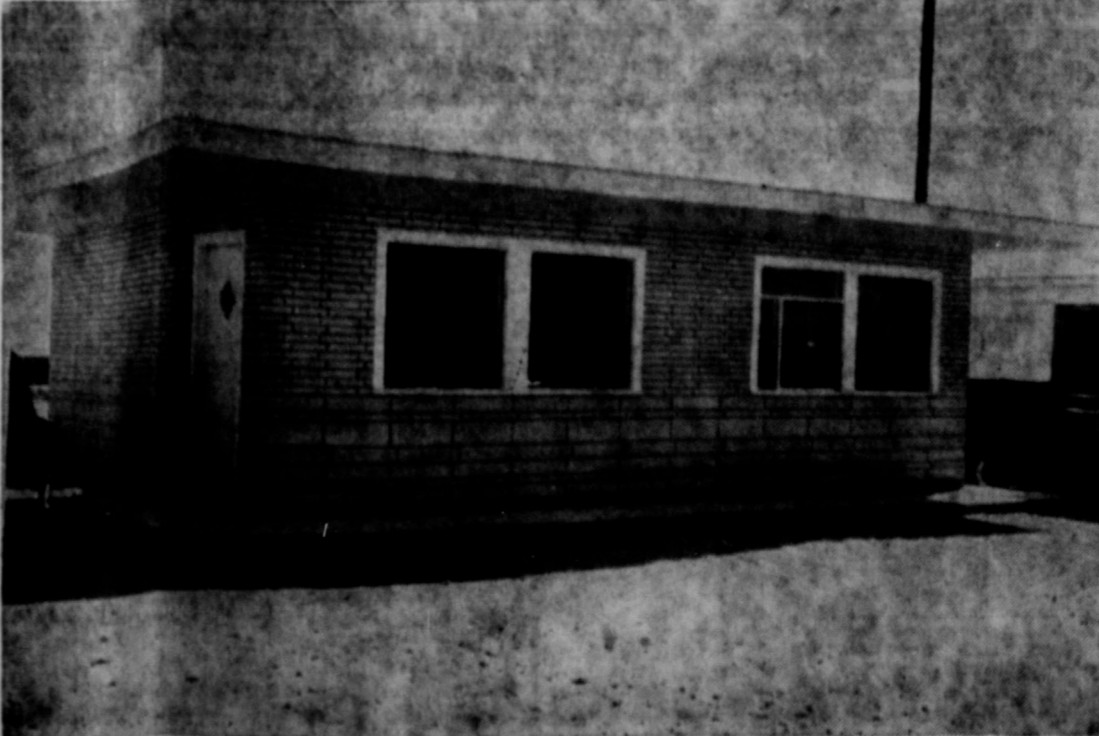
DANNA'S DRIVE INN will stage a formal opening Saturday from 1 to 4 p.m. Free coffee and Donuts will be served to all who attend and free balloons for the children. The new building was completed last week. Mr. and Mrs. Troy Davis own and manage the Drive Inn.
