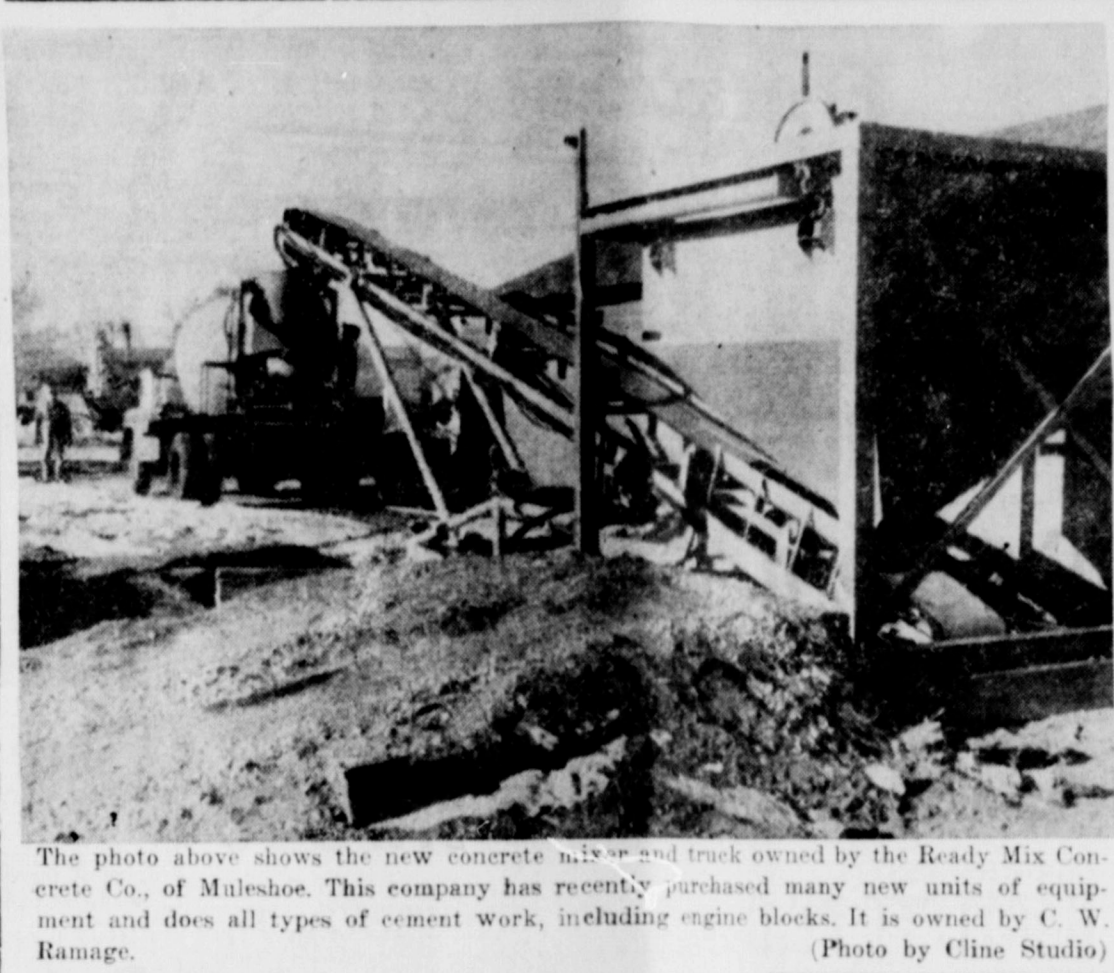
The photo above shows the new concrete mixer and truck owned by the Ready Mix Concrete Co., of Muleshoe. This company has recently purchased many new units of equipment and does all types of cement work, including engine blocks. It is owned by C. W. Ramage. (Photo by Cline Studio)
