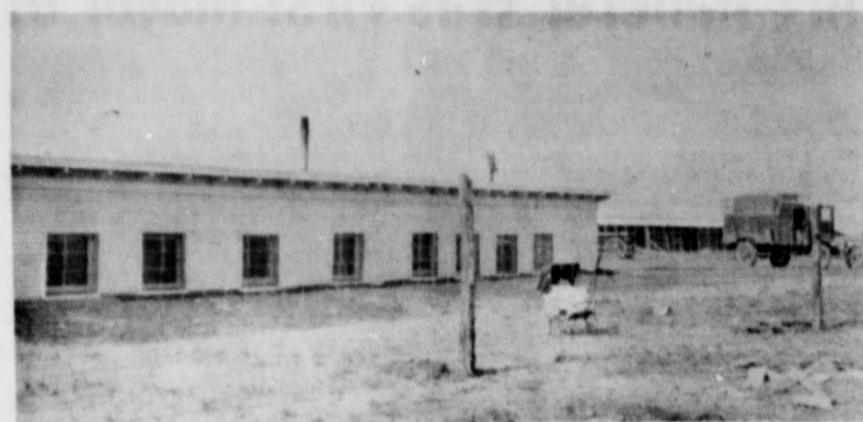
THIS WEST TEXAS BUNGALOW was built by C. V. Harmon to house his family in 1924. The truck in the background is a 1917 Model T that was used for hauling wheat as well as the source of the family's transportation. The baby carriage center was typical of those used for the babies of the growing families. The house was located 3 miles northeast of Amherst, and was a half dugout which was roofed and had windows on all sides.
