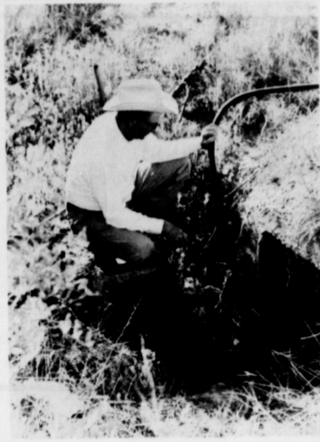
THIS WELL, located west of town between Highway 70 and Halsell ranch, was dug for irrigation purposes, back in the early 20's by Mr. Halsell. In order to pump the water, a 20 foot deep pit was dug and a centrifugal pump set, right on top of the water and the water pumped by a diesel engine out of the pit through the discharge pipe. In the first picture T. V. "Red" Murrell stands near pit used as a cooling system for the pumps. In the center photo, Murrell stands looking over the discharge pipe leading from the bottom of the well. In the last picture, Murrell is shown down in the 20 foot deep cement pit. Incidentally, T. V.'s brother, Hohmy, was the last person to operate the well back in 1936.
