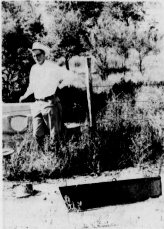
THIS WELL, located west of town between Highway 70 and Halsell ranch, was dug for irrigation purposes, back in the early 20's by Mr. Halsell. In order to pump the water, a 20 foot deep pit was dug and a centrifugal pump set, right on top of the water and the water pumped by a diesel engine out of the pit through the discharge pipe. In the first picture T. V. "Red" Murrell stands near pit used as a cooling system for the pumps. In the center photo, Murrell stands looking over the discharge pipe leading from the bottom of the well. In the last picture, Murrell is shown down in the 20 foot deep cement pit. Incidentally, T. V.'s brother, Hohmy, was the last person to operate the well back in 1936.
