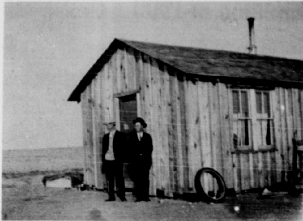
The first house in Earth was built in April or May of 1924, even before the Haisell Hotel, which was started in August of that year. The house was built by Loyd Cupp and was 2 rooms, unpainted and had only partial partitions, and no sealed ceilings or walls. It was later occupied by the Cearley family. It is still standing today two blocks northwest of its original location, back of the Steak House. Sam and Carl Cearley stand before the house.
