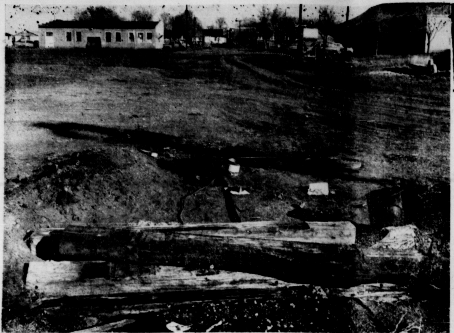
Here is one unit of the crude, primitive, expensive pump and dump cesspool system that served an enrollment of 729 students this year. Another cesspool may be seen at upper right hand towards corner of High School building.
