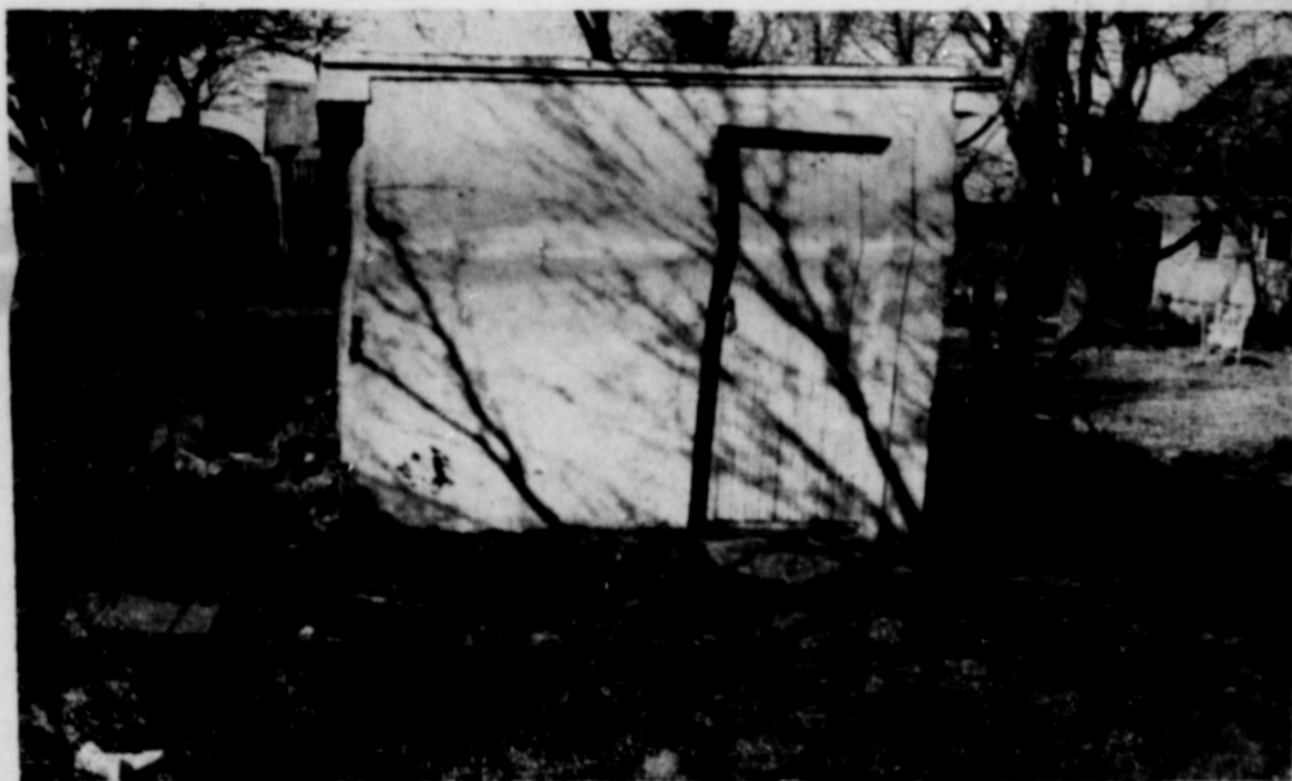
This small building houses the pressure pump system which furnishes water to a student population almost equal to that of Earth. What kind of fire protection does this water system provide? Remember, the electrical system is the first thing to go out in the event of a fire.
