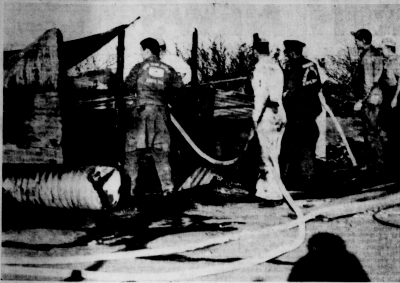
EARTH FIRE DEPARTMENT roared eight miles out to the Paul Templeton farm Monday to extinguish a burning chicken house. The small building was destroyed by the time they arrived, but they prevented possible damage to other buildings. A south wind carried the sparks into an open field. A wind from any other direction would have seriously endangered either barns or dwellings. (News Photo)
