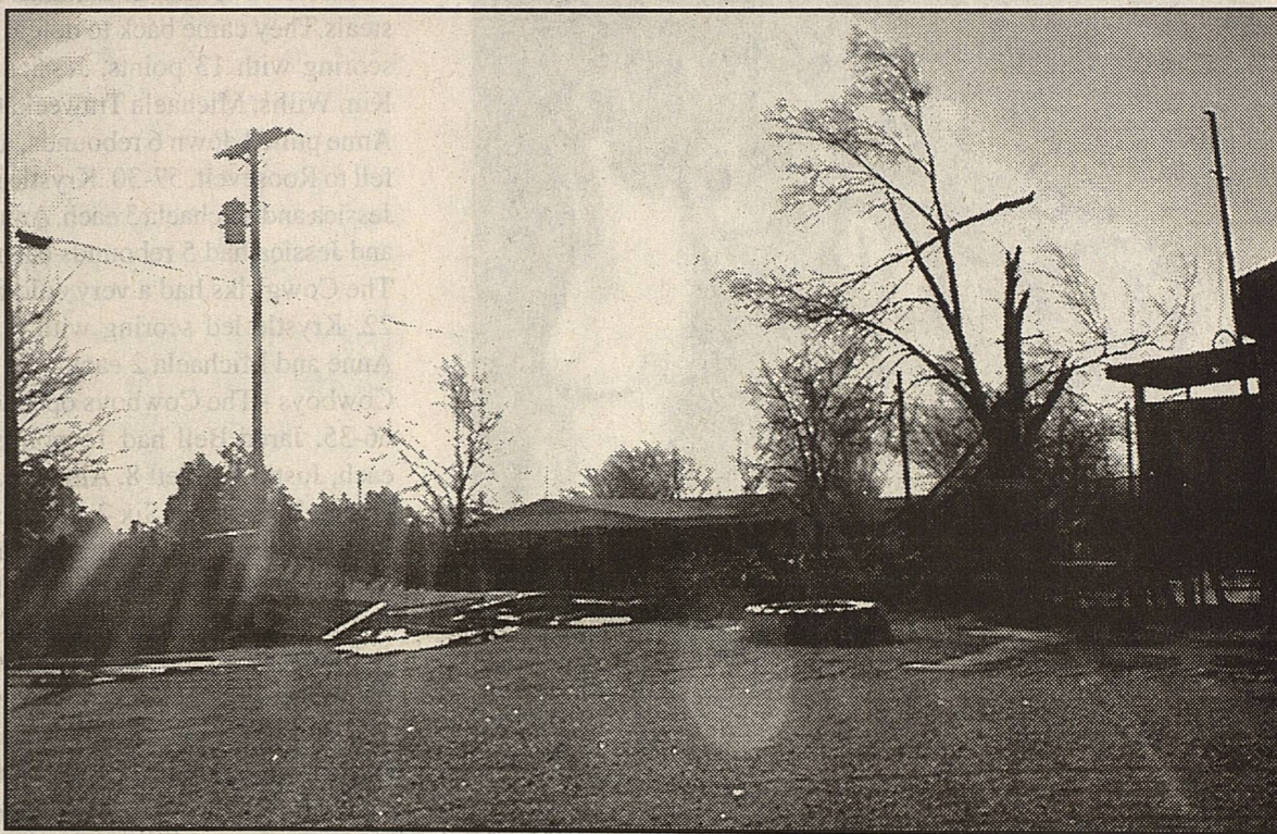
Debris from the roof of the mobile home at far right is shown piled against fence at left. Note broken tree limbs at side of home
