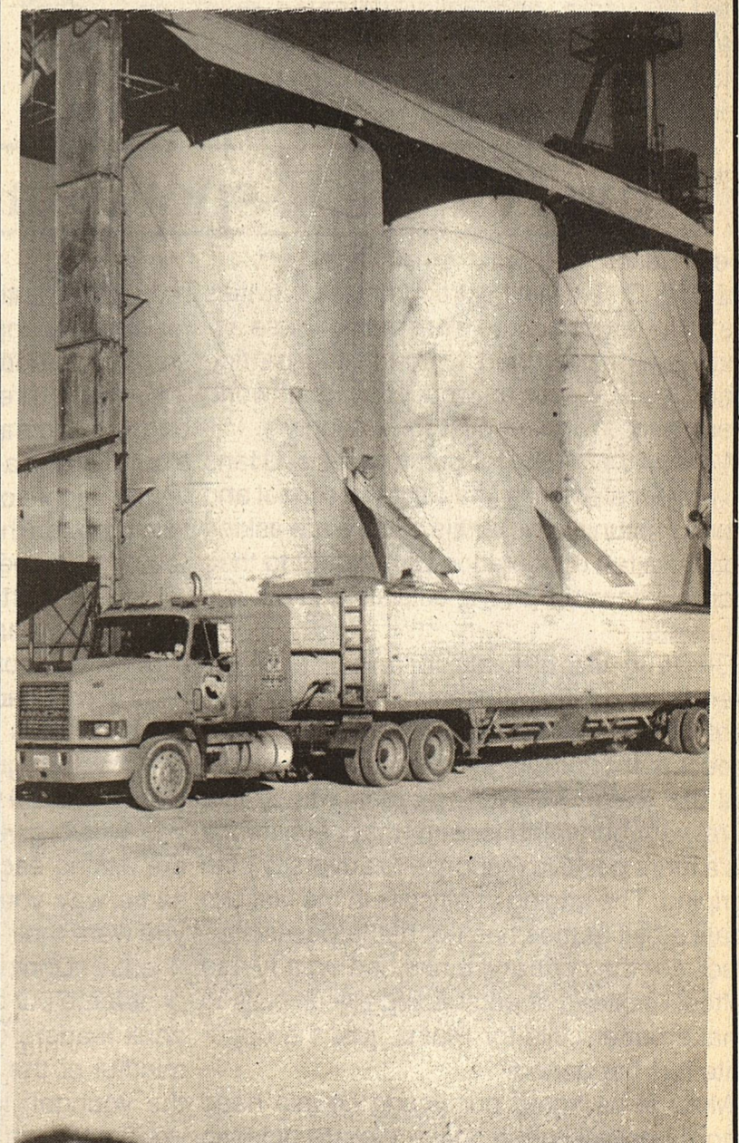
The grain truck shown loading milo at the Goodpasture elevator is a familiar sight there and at the Seller's two storage sites. Approximately 100 million pounds of grain sorghum were delivered to the two facilities, the largest crop in a number of years. Dare Walker at the Goodpasture elevator reported workers were loading over twenty semi-truckloads daily last week. The large milo crop resulted when many acres of cotton were destroyed by either hail or high winds.
