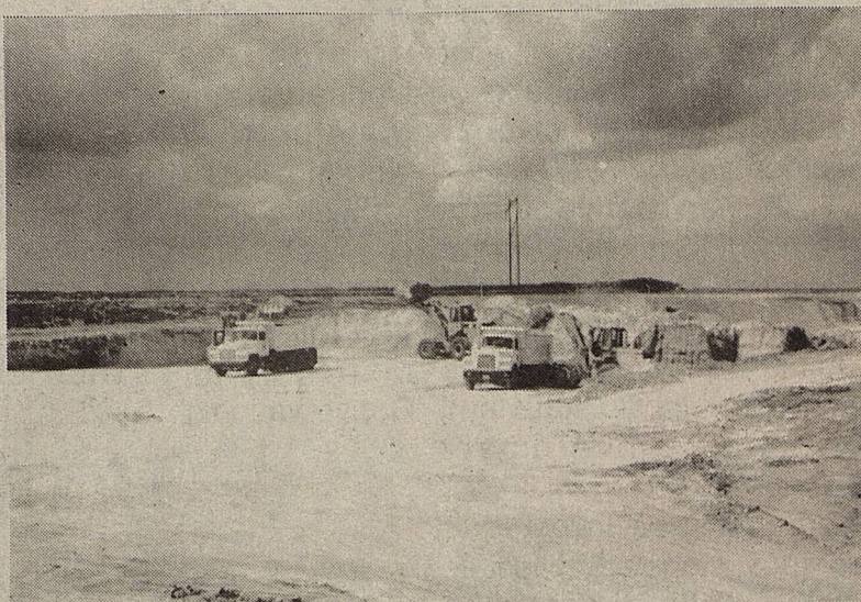
DIGGING DIRT, MOVING IT TO NEXT LOCATION
