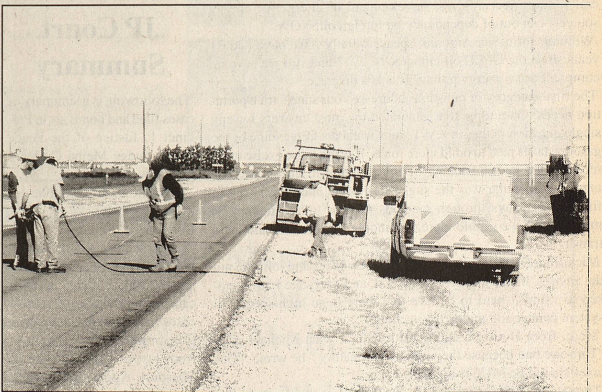
Pct. 1's Woody Lindsey and Galen Ford discuss plans for improving safety of the 1780 & 213 highway intersection, above, and TxDOT crew lays down 'Rumble Strips' to alert drivers to stop sign at intersection.
