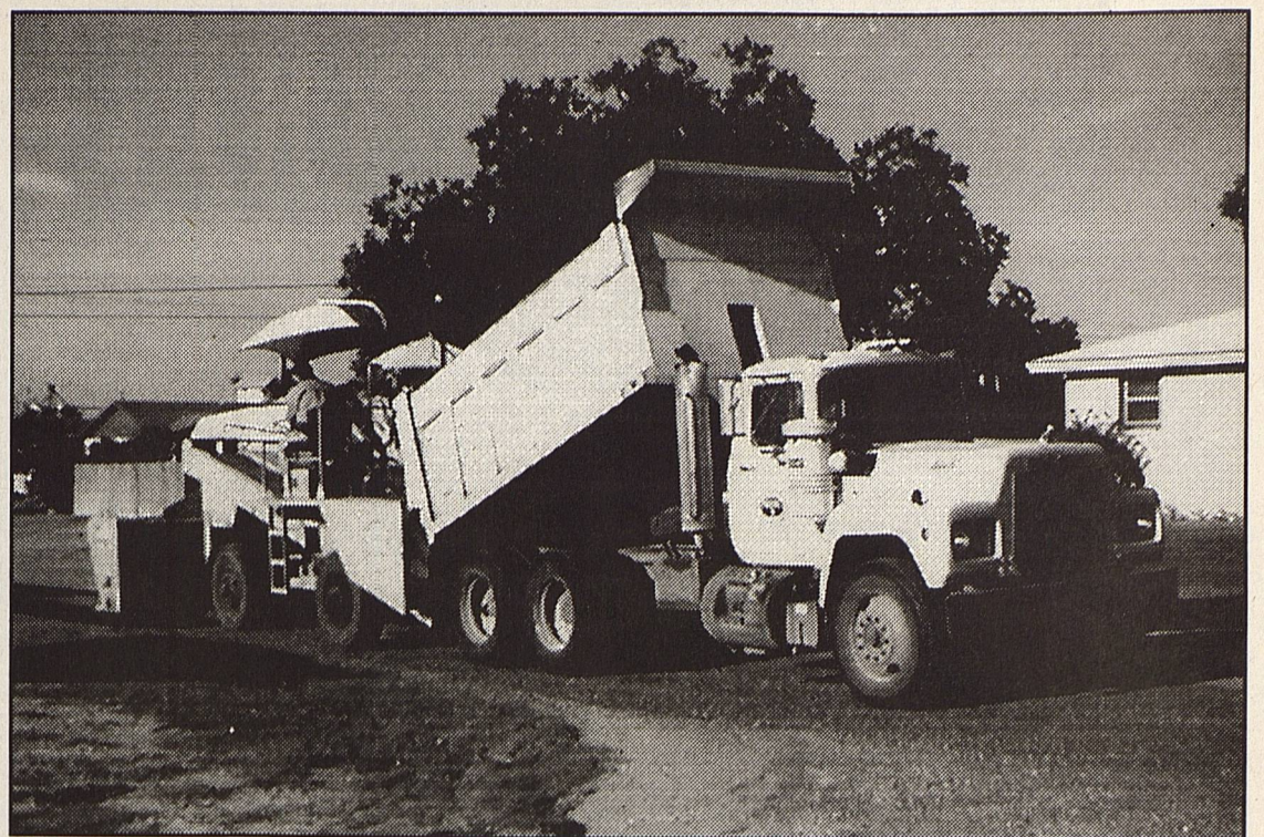
Precinct 3 and 4 personnel were busy last Thursday applying a new seal coating to Avenue B at US 82/380 to First Street. The road repairs were then extended to the county airport. The new surface should help alleviate normal problems this winter.
