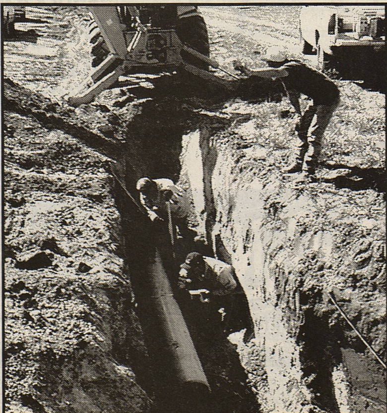
City employees prepare to make last connection just west of town
