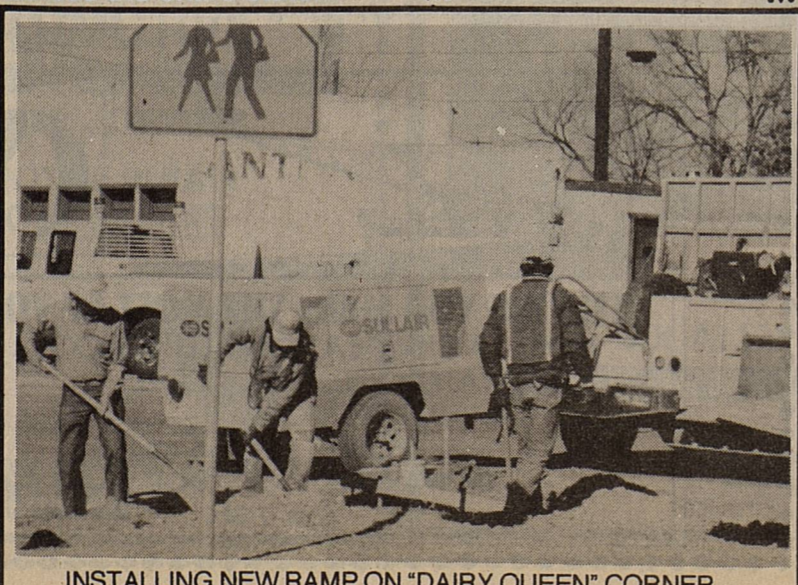
INSTALLING NEW RAMP ON "DAIRY QUEEN" CORNER
