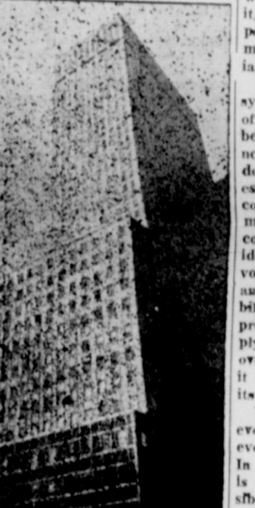
SCENE - STEELER - Sparkling new addition to the Manhattan skyline is this 45-story Sohoany Motel Building, first and world's largest stainless steel skyscraper. Recently dedicated, the building has a "cor-nerised" in which is sealed a three capsule, holding messages from President Eisenhower, Governor Marjames and Mayor Wagner, as well as copies of New York newspapers and documents detailing construction of the unusual building.
