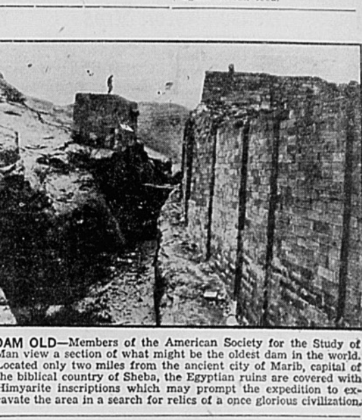
DAM OLD —Members of the American Society for the Study of Man view a section of what might be the oldest dam in the world. Located only two miles from the ancient city of Marib, capital of the biblical country of Sheba, the Egyptian ruins are covered with Himyarite inscriptions which may prompt the expedition to excavate the area in a search for relics of a once glorious civilization.
