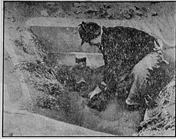
DUST STORM AFTERMATH —Albert Brabander digs out a culvert on his father's farm near Shawnee, Kan., after recent dust storms swept over the land. When the winds abated, loose soil like this was deposited like minor snowdrifts over many Midwestern farms, causing damage to crops which is still not fully estimated. Weather Bureau and Department of Agriculture officials admit that nature may be setting the stage for storms which could match the disastrous "Dust Bowl" days of the Thirties.
