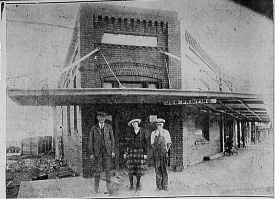
Slatonite, And Staff 25 Years Ago
