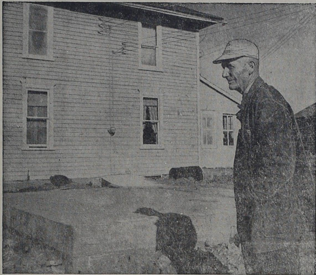
SURVIVAL INSURANCE looks like an ordinary concrete slab at the home of Don S. Trow near Albany, Wis. But beneath the slab is a $1,500 reinforced concrete shelter which the 68-year-old farmer ordered built for himself and his wife. Trow got the shelter plans by writing to Box Home Shelter, Office of Civil and Defense Mobilization, Battle Creek, Mich. (Wisconsin State Journal Photo)
