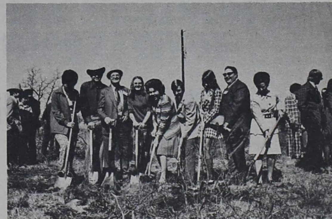
GROUND BREAKING —Digging in to assist with the Texas 4-H Center groundbreaking ceremony at Lake Brownwood recently were these adult 4-H leaders and youth from Extension District 2. Pictured (left to right) are Mrs. Dewey Drennan and Mr. Drennan of Welch, in Dawson County; John I. Bowling of Hale Center; Jane Drennan of Welch; Mrs. Catherine B. Crawford, District Extension Agent (home economics) at Lubbock; Steve Stanley, 4-H youth from Levelland; Rene Nelson, Brownfield 4-H girl; and Mr. and Mrs. Floyd Terrell of Plainview. Mrs. Terrell was a featured speaker. Construction on the $1.375 million Center is getting underway on a scenic 78-acre site adjacent to Lake Brownwood. T. Louis Austin of Dallas, chairman of the Texas 4-H Youth Development Foundation, presided at the recent Brownwood ceremony. Construction of the Center is expected to require about a year.
