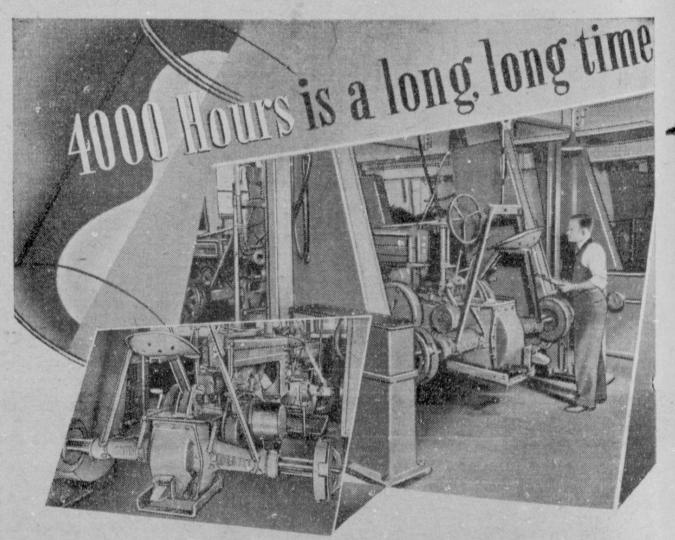
FOUR thousand hours is a long time to keep a tractor operating at high speed, at peak load. But, that is the break-down test new models of John Deere Tractors must pass before they are ready for production-4,000 hours without failure.
