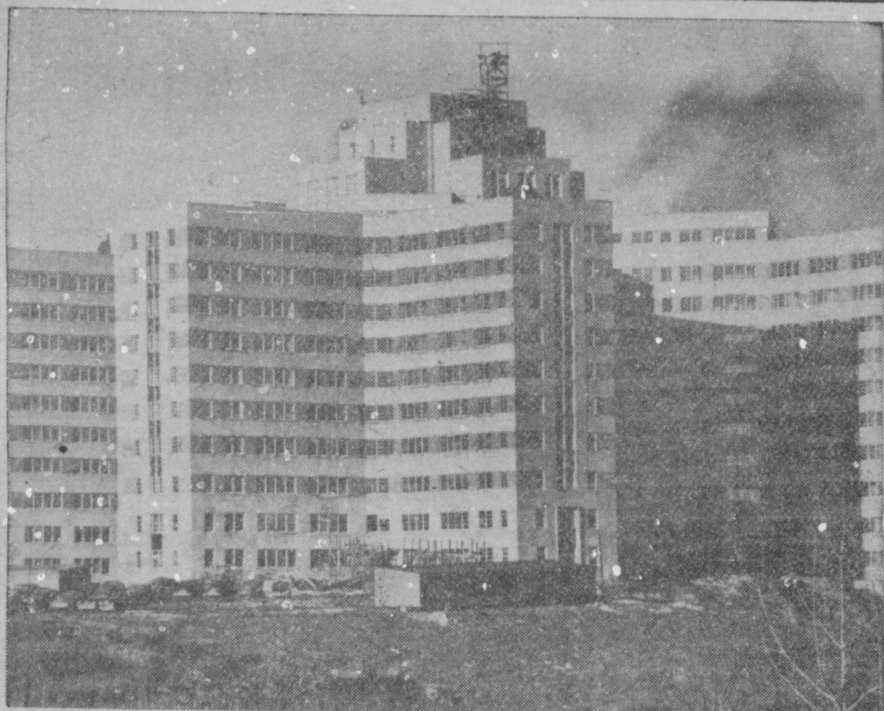
NEARING COMPLETION —The outer shell of the new Veterans' Administration Hospital, in Albany, N.Y., is almost finished. The 14-story building, of fireproof construction, will have a capacity of 1000 beds when it's ready for the first patients.
