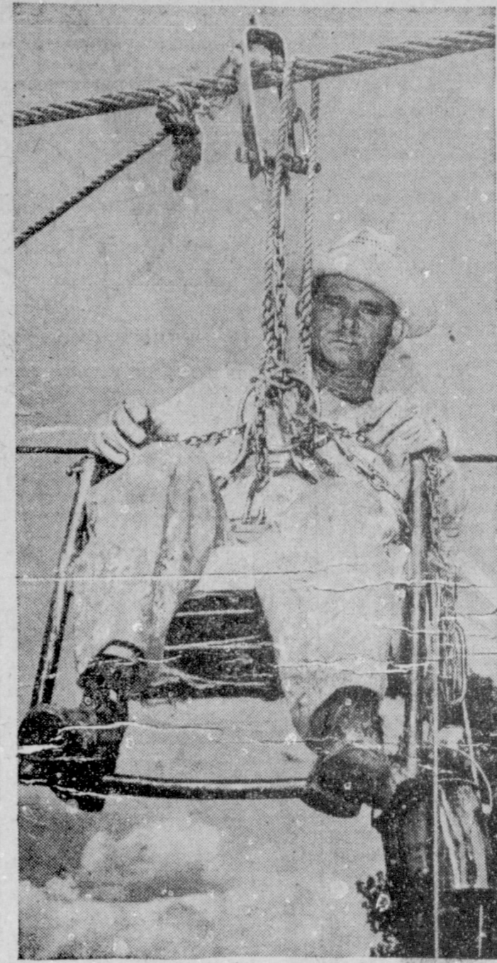
Invented by members of Lone Star Gas paint crew this boat-swain's chair enables them to paint pipeline suspension bridge rods in less time than they used to require. It was designed primarily for the safety of the painter.
