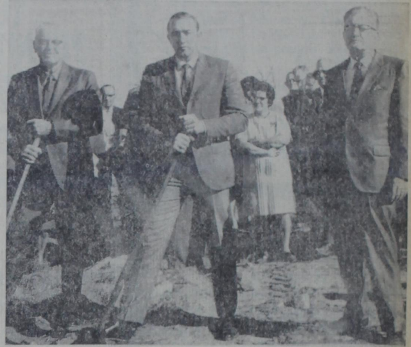
GROUNDBREAKING CEREMONY—L. J. Collins, chairman of the First Baptist Church building committee; Franklin Cox and Rev. Vic Allen pose in acts symbolic of the beginning of construction on the new First Baptist Church which will replace one lost by fire last October. The picture was taken during a special service at the site Sunday at 2 p.m. attended by a large number of the congregation.
