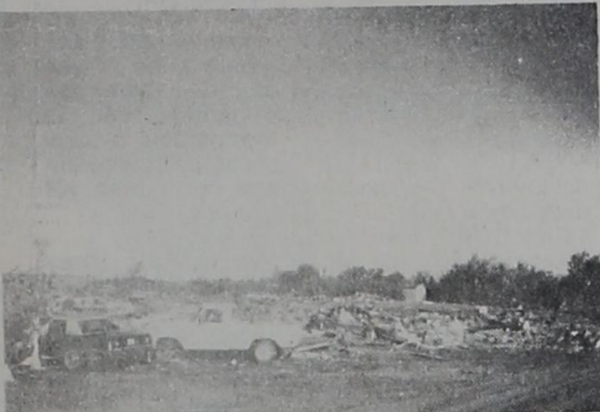
TRAILER PARK After Sweetwater tornado, April, 1986. Pickups were not there during the storm.
