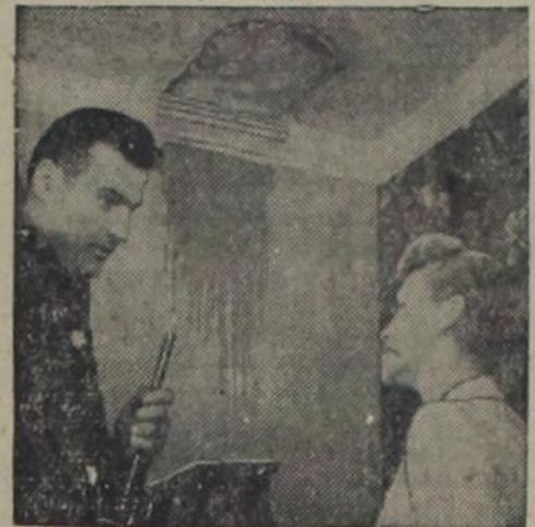
Plumber tells housewife leaking soil pipe is danger to family's health and that wall must be torn out for repairs.
