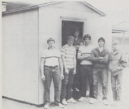
THE ADVANCED Woodshop students of Muenster High School are building an 8'x10' storage building as a class project. Students learn the principles of residential construction beginning with sill and joist construction for the floor. Wall framing and rafter work follows with the roof being decked and shingled. Masonite siding is applied to the exterior wall and trimmed with redwood.
