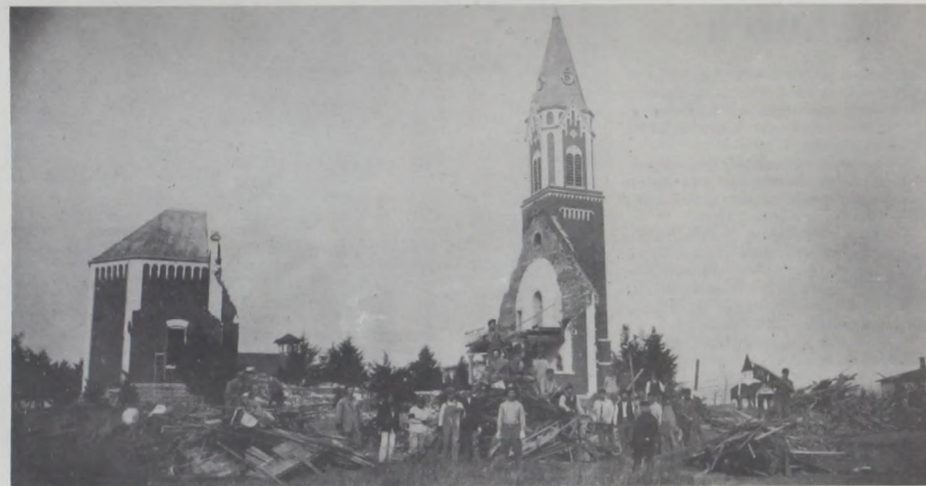
debris to the church ... the church which had been completed the previous January and which had been the pride and joy of all.
