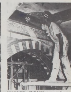
WORKER CLEANS the walls and ceilings before painting begins.
