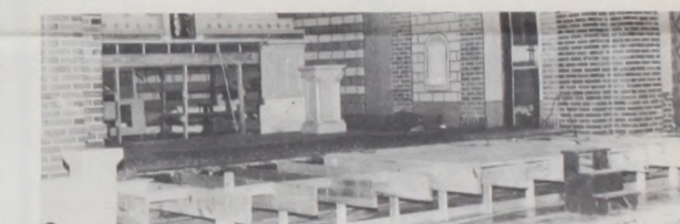
THE FLOOR of the sanctuary being extended and the altar table removed.
