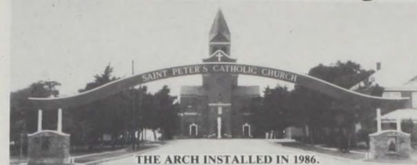
THE ARCH INSTALLED IN 1986.
