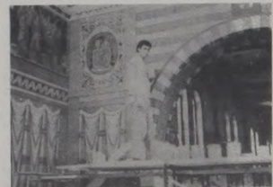
MIKE BROWN repainting damaged wall in 1978.
