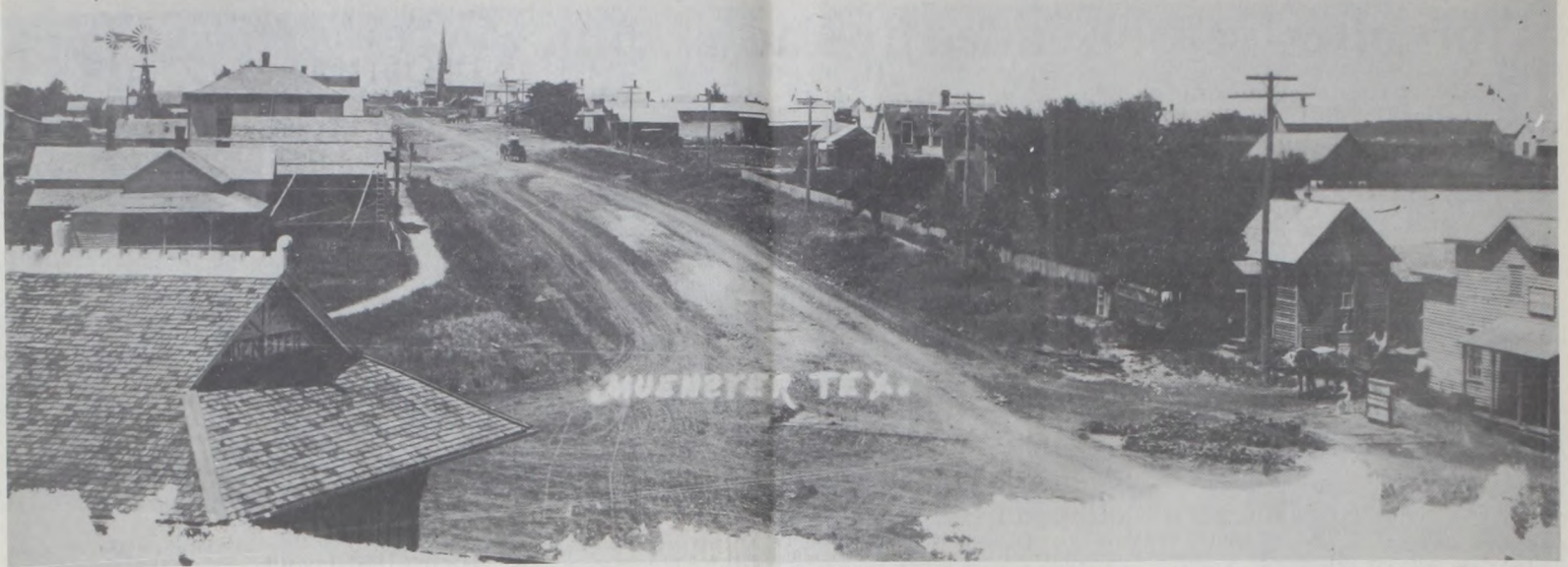
MAIN STREET, MUEENSTER , taken about 1920, from south of the railroad tracks. The roof to the left of the picture is the old depot. Next to it is the Henry Stelzer home. The large, two-story building, with the wood windmill, is the old Knights of Columbus Hall. At the far right is the old Waples Painter Lumber Company, Tony's Seed and Feed Store is now in that building. Beside the building is a wagon hitched to a team of horses with a load of lumber. Charles Reiter lived in the house next to it before moving to Kerrville. The two-story house is
