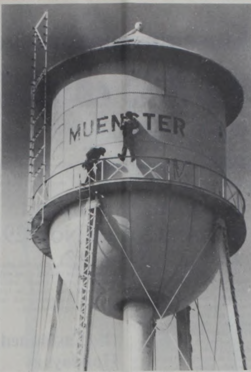
WORKMEN FROM MIDWEST TANK COMPANY of Kansas are busy now, when weather allows, sandblasting and preparing the Muenster water tower for a new coat of azure blue paint. Refinishing is planned for the outside and supporting structure only. Janie Hartman Photo
