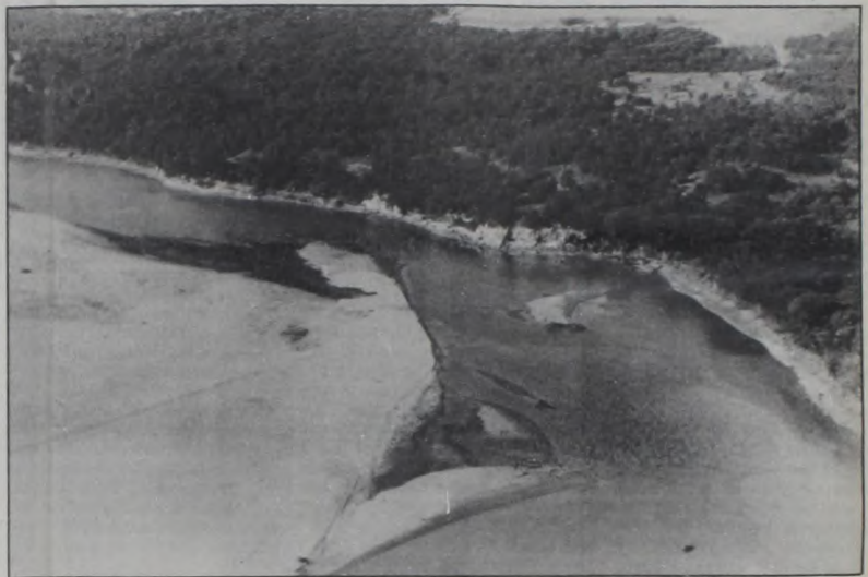
SITE FIVE , previously known as Rock Bluff on the Red River, as seen from the air and the northwest, is the favored location for the proposed new bridge by most Muenster and Saint Jo area residents. Besides being centrally located for the area, the bluffs offer a
