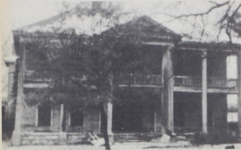
THE OLD BELLAH HOME before its remodelling and restoration...
