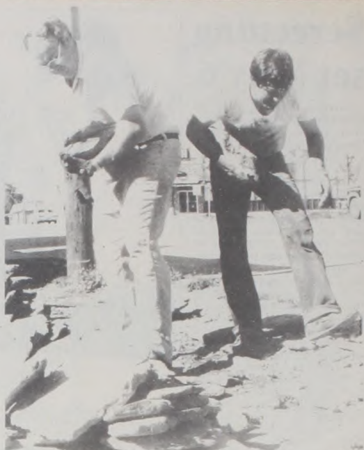
DOING HARD TIME, Charles Coffey (left) and Gary Fisher select and move rocks to complete a section of wall bordering a flower bed at the nearly-complete Elder's Park downtown. Photo by B. J. Fenton
