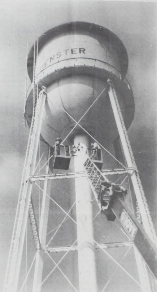
A sizeable project was needed to repair two tiny drips in the city water tank. It involved moving a crane from Irving for the short job and draining the tank to relieve pressure. Service was continued by closing the tank's intake valve and pumping continuously through the mains. Janie Hartman Photo
