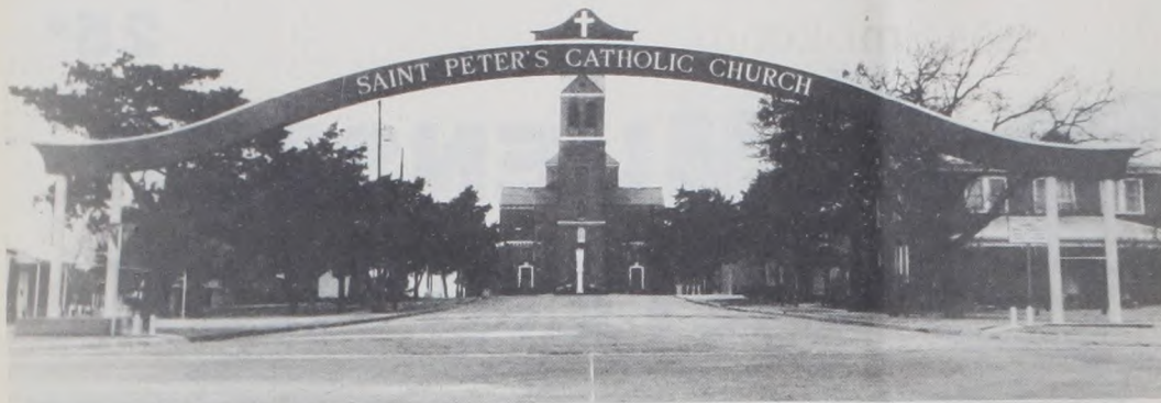
Lindsay's Arch, forming a stately entrance to parish grounds and St. Peter's Catholic Church is the newest and most outstanding addition to the community. It is 80 ft. wide, spanning the street beyond both curbs, and is made of 5000 lbs. of steel. It was built by JAW Construction and is well equipped with electrical connections. Special spaces are planned inside the supporting pillars for two statues, one of St. Isidore, patron of Farmers, the other of St. Peregrine, patron of cancer patients. There will also be a large plaque to list Mass schedules and parish announcements. The arch is a memorial given by an anonymous donor. Janie Hartman Photo
