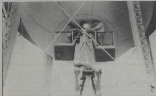
A SIZEABLE PROJECT was necessary to eliminate two tiny drips at the city water tank last Friday. It involved moving a crane from Irving for the comparatively short job and draining the tank to relieve water pressure. Water service was continued by closing the tank's intake valve and pumping continuously through the mains, however, pressure was low. David Fisher and Mike Sturm are shown in the crane's cage welding on the repair patches.
