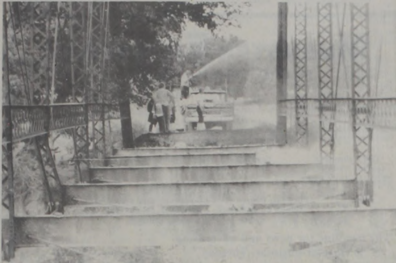
THIS STEEL SKELETON is the remains of a bridge fire of unknown origin about noon Friday on Elm Creek near Reed Cemetery two miles southeast of Myra. All of the floor was burned and some of the frame was warped by heat. Firemen of Myra and Muenster confined the fire's spread to an area of about one acre.
