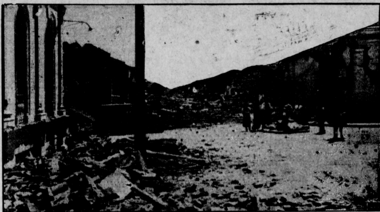
CONCEPCION, CHILE—Radiophoto—A scene of desolation in this city in South Chile which was virtually wiped off the map by the earthquake on Jan. 24. Seventy per cent of the buildings were razed and the dead were numbered at more than 2,500. Concepcion is Chile's southern capital.
