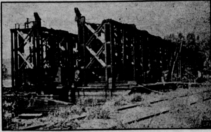
PRAIRIE DU CHIEN, WIS. —One of the most unique type of bridges in the world is the pontoon bridge of the Milwaukee railroad over the Mississippi River at Prairie du Chien. Only two of its kind are known to exist in the world. Above is a view of the 230 foot floating pontoon of the bridge as it was hauled up on the banks of the Mississippi River at Prairie du Chien for repairs. Boats on the river will be forced to use the west channel of the river since an immovable piling has been installed across the river where the pontoon originally stood.
