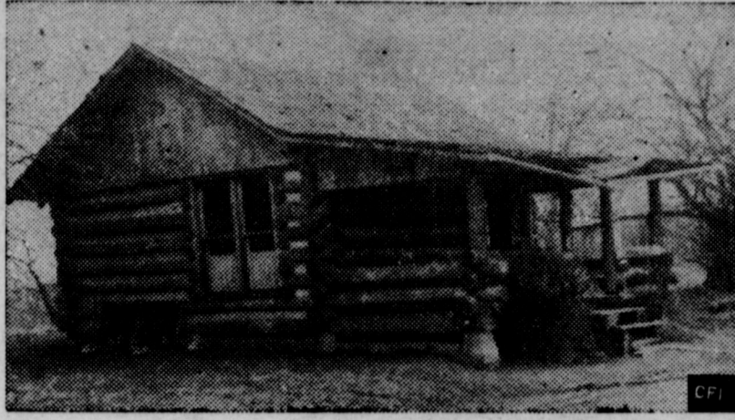
The above one room log cabin of Dr. Perry Baldwin is the only real rural dental office in the midwest. It is located 18 miles from Jasper, Ind., the nearest town of any size. Dentist Baldwin uses a foot-powered drilling machine and works by the light of a coal oil lamp. He has more patients than he can handle.
