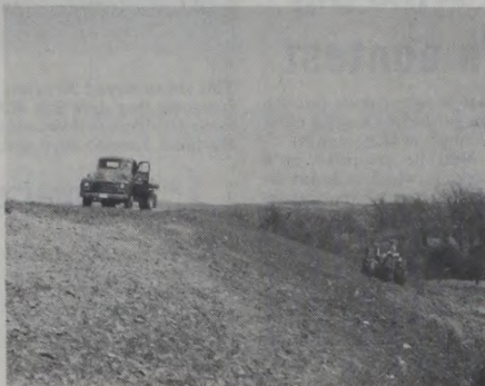
SCS Photo Here's how Bermuda grass was sprigged on the emergency spillway of Site 23 Reservoir on Clear Creek. A cable, barely visible in the picture extends from truck to tractor to keep the tractor from turning over. Picture taken March 23, 1962.
