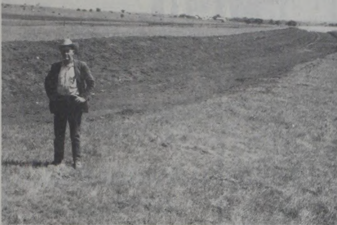
Soil Protection. This photo, taken June 1, 1967, shows Ed Cler in the channel of a diversion terrace recently completed on his farm. The diversion protects cropland below.
