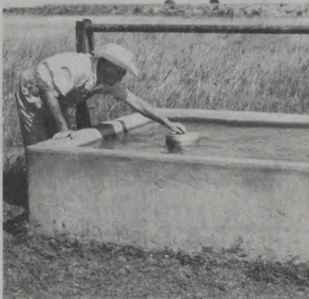
SCS Photo This picture, taken in Aug. 1968, shows Tony Waterscheid adjusting the float valve on his watering trough. When he constructed the new pond in the background he installed a steel pipe through the dam and connected it with 260 feet of plastic pipe leading to the concrete trough. The system provides a good quality of fresh, clean water for livestock of two pastures.
