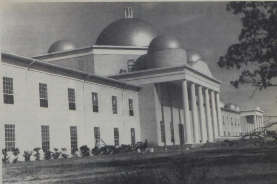
The "capital" in Forestburg was designed by an Australian architect according to Maharishi's specifications. All of the Transcendental Meditation Centers have domes on the exterior. This particular structure has 15 gold domes on the outside, five on each end
