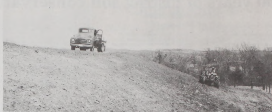
Watershed Clear Creek-Trinity springing emergency spillway with common bermuda grass - 1962
