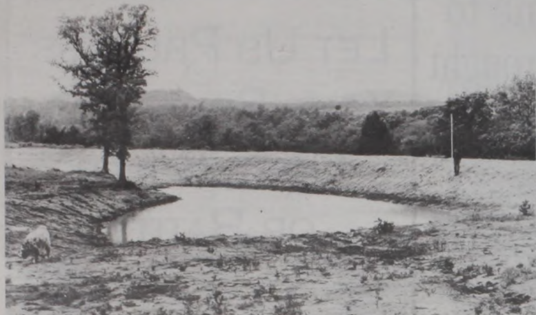
Bill Harris, last years Zone III conservation winner continues the practice on his farm north of Saint Jo. The diversion and grade stabilization structure should help control erosion and run off so the damaged can be dozed and repaired.
