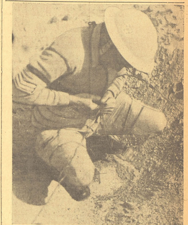
MUST GO ON —It's important that communications remain open, in North Africa. Here, British signaller in full view of enemy quickly splices broken cable severed during temporary stand by Rommel.
