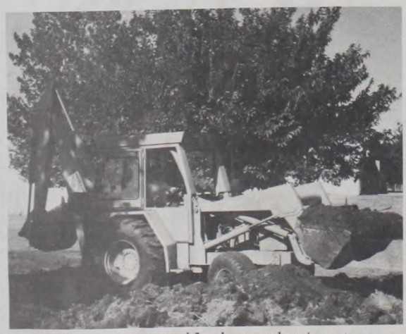
Backhoe prepares ground for playground equipment. (See related photos page 2)
