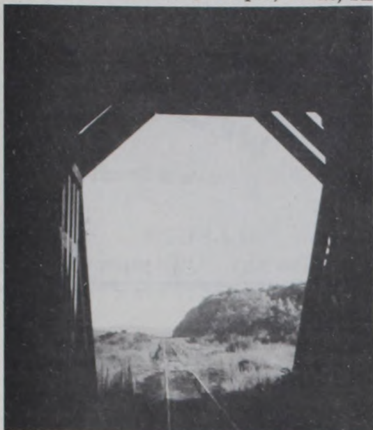
Quitaque Tunnel - the only remaining tunnel in the state.
