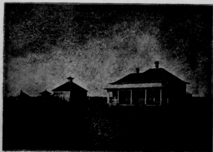
ROREDALE, RESIDENCE OF J. M. CONN
