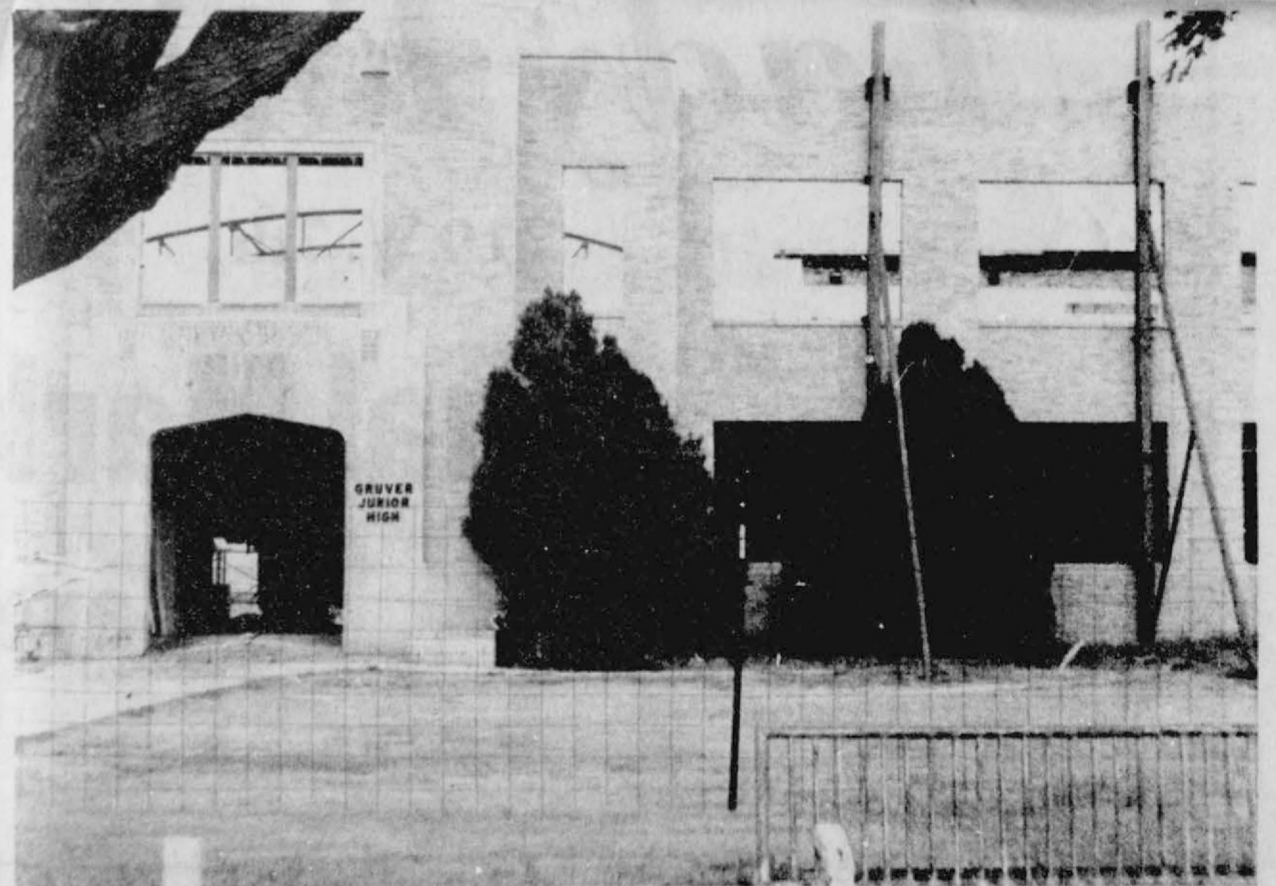
Work underway at Gruver Junior High.
