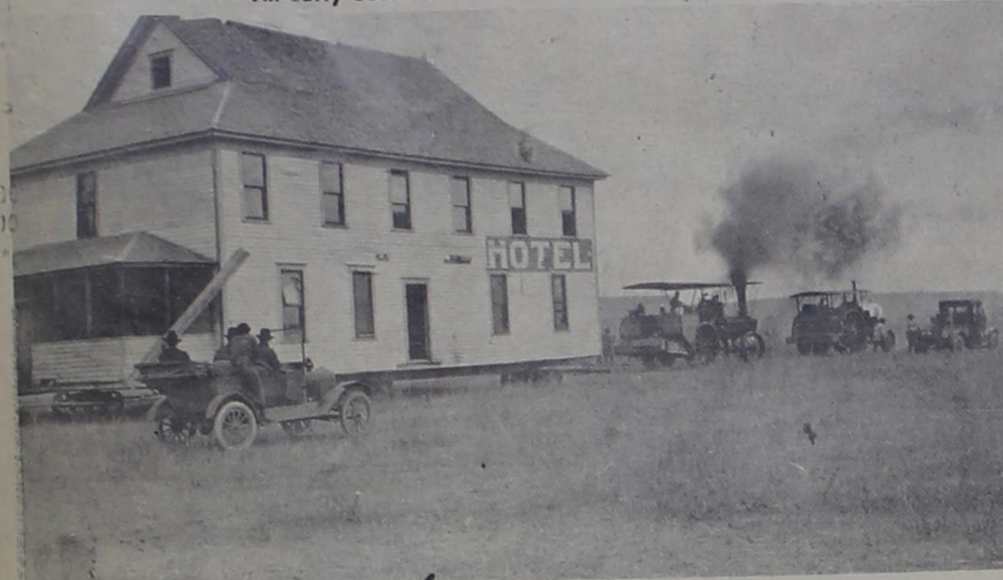
The Hansford Hotel was moved to Spearman along with many other buildings
