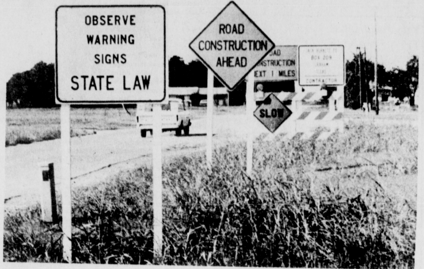
SIGNS OF PROGRESS - Texas Highway Department workers this week put up signs on Pacific announcing improvement work they will be undertaking over the next
