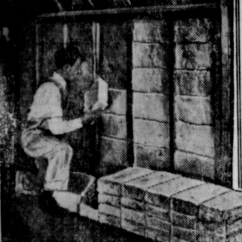
An important phase of America's 1938 building program is home insulation with mineral wool. Because of the economy and the ease with which it may be used on both new and old homes, architects and builders recommend complete insulation with mineral wool. At upper left, workmen are placing four-inch bats of fire-proof mineral wool between sidewall studs of a new home. At lower right is demonstrated method of filling sidewalls of old houses with mineral wool for year round comfort and economy.
